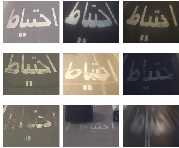
Fig. 4: “Caution Text” class with different qualities: First row includes “Excellent” quality markings. The second row includes “Fair” quality markings. The third row includes “Poor” quality markings. All of them are selected from the PRSM dataset [6].
