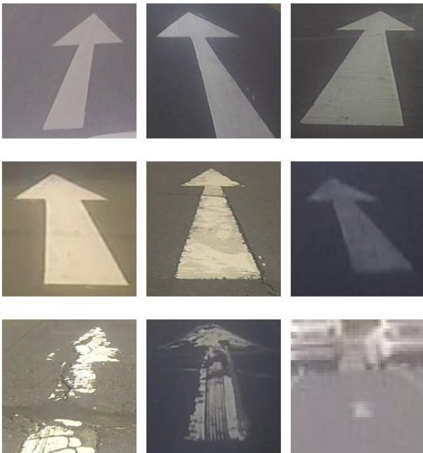
Fig. 3: “Forward” Symbol class with different qualities: First row includes “Excellent” quality markings. The second row includes “Fair” quality markings. The third row includes “Poor” quality markings. All of them are selected from the PRSM dataset [6].
