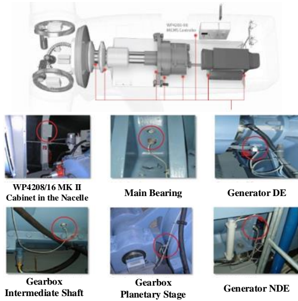
Fig. 14: Location of vibration sensors of MAPNA WT condition monitoring system.
